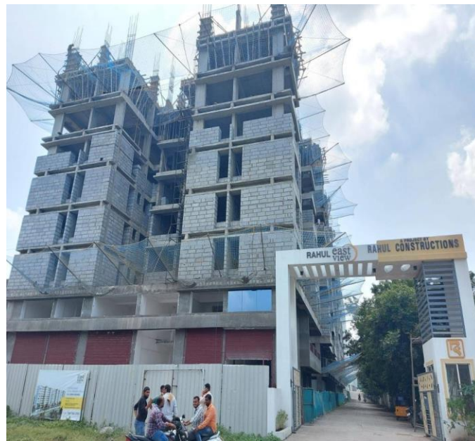
Fig 6: Site Entry & Exit photo
